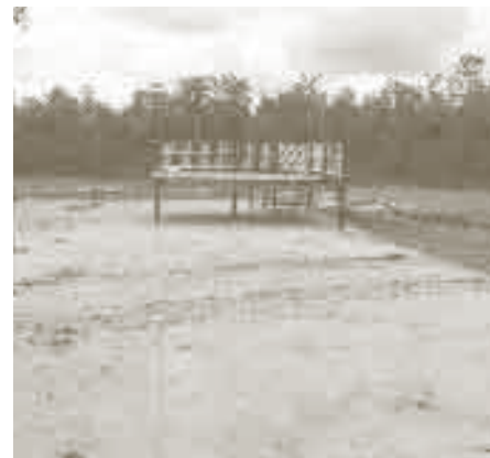
Little remained of some buildings after flood waters had passed through
